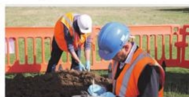
• Workers studying soil from a trial pit
